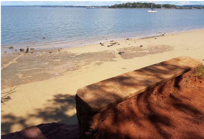
Community Hall, Jetty, Steps, Coochiemudlo Isl (AHS, 2017).
