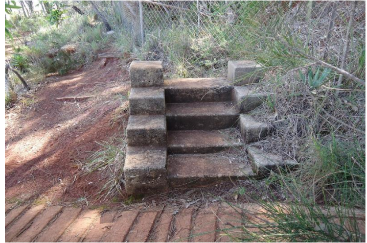
Community Hall, Jetty, Steps, Coochiemudlo Isl (AHS, 2017).
