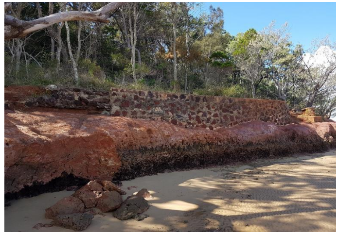
Community Hall, Jetty, Steps, Coochiemudlo Isl (AHS, 2017).
